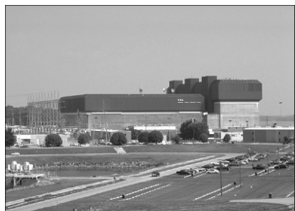
Titelbild: Browns Ferry Nuclear Power Station. Three Boiling Water Reactors with a total capacity of 3,300 MWe net. Unit 1 was reconnected to the grid in 2007 after a lay-up operation since 1985 (Courtesy: Tennessee Valley Authority TVA).
